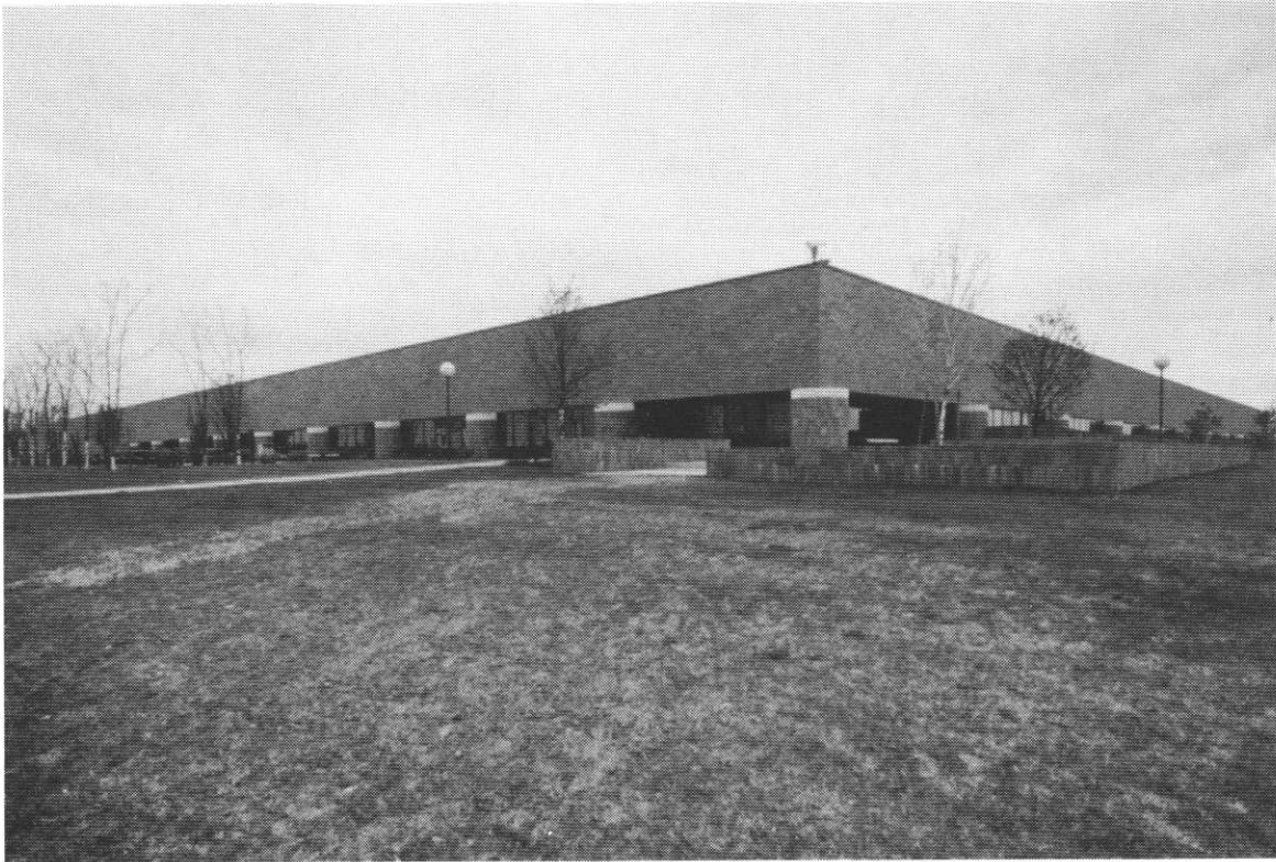
DIGITAL Facility, Hudson, Massachusetts
